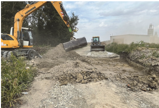
Figure 10. Mixing of wood ash and crushed material from excavation [32]
