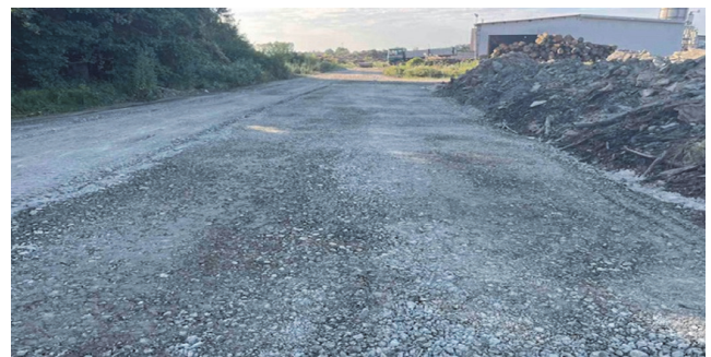
Figure 8. The constructed unbound pavement of the internal road made of crushed stone [32]
